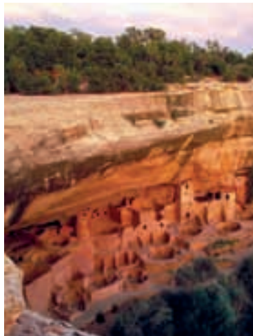
Cliff Palace, the largest dwelling at Mesa Verde, may have housed 250 people.
